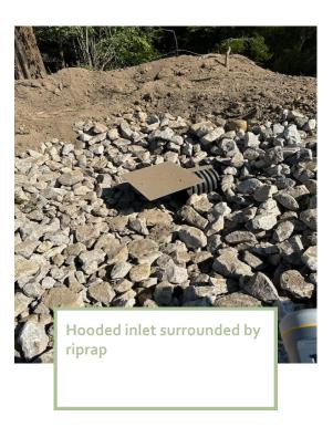
Typically supplied by quarries, riprap has angled edges that lock together and help to hold the stone in place.
